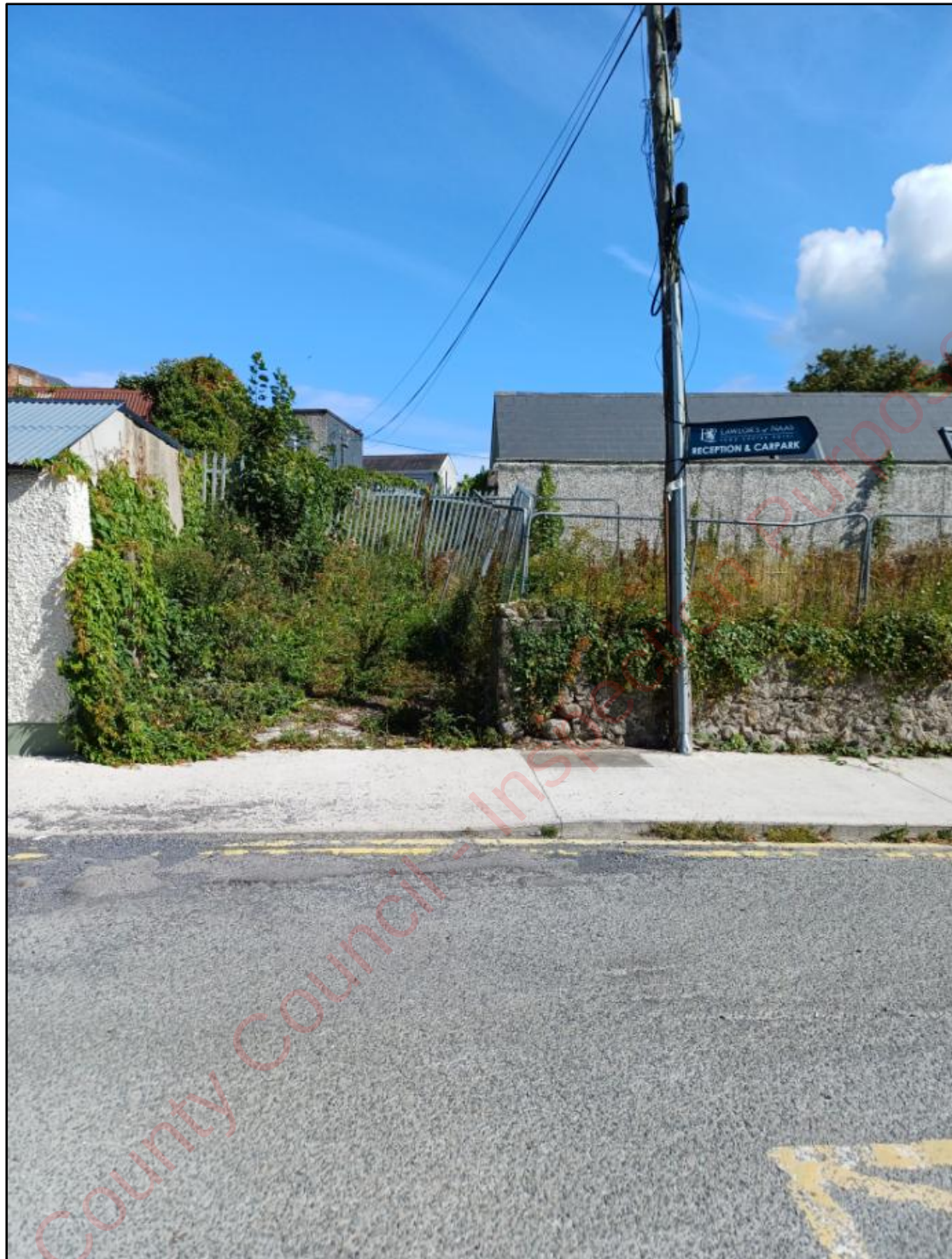
Fig 10: Site inspection photo.
