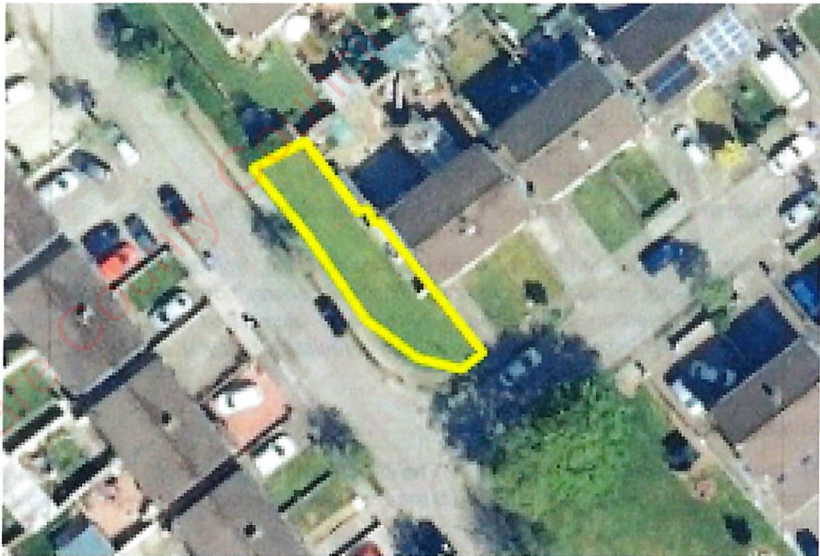
Figure 2: Aerial view of site (subject site outlined in yellow)
