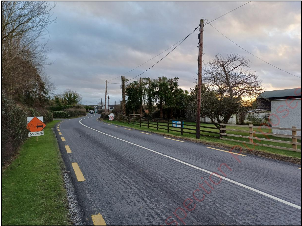
Figure 6: Site Inspection Photo
