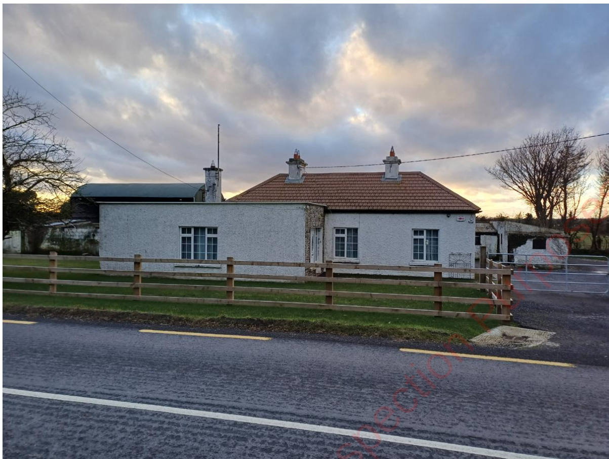
Figure 7: Site Inspection Photo
