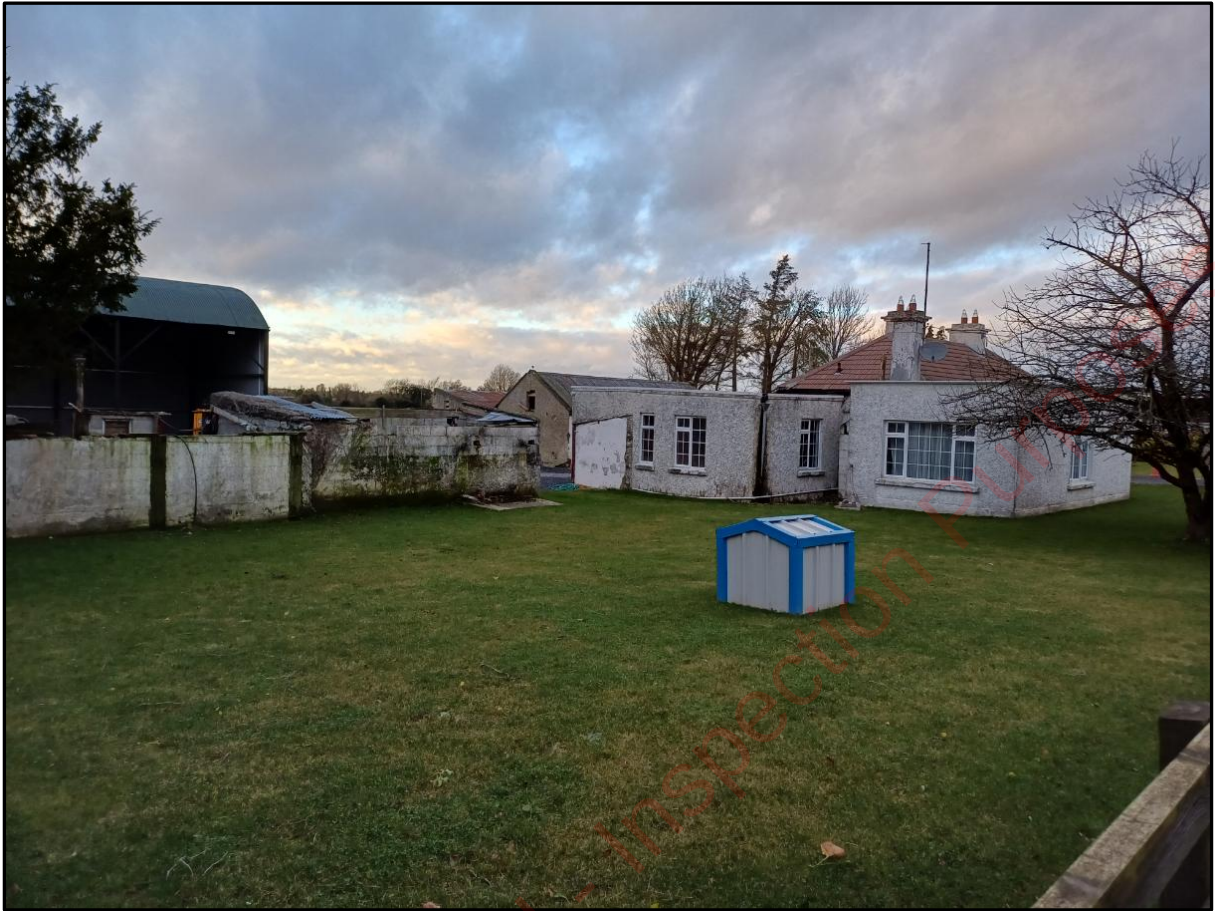
Figure 4: Site Inspection Photo
