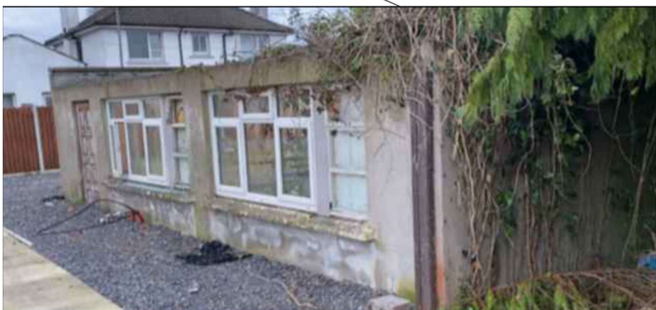
Image 'A' of shed before renovations.
