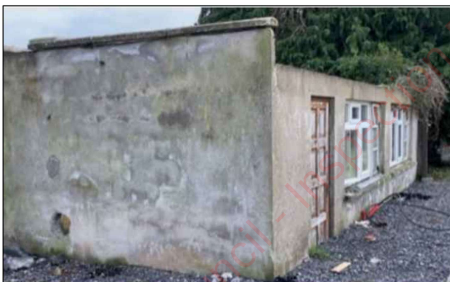
Image 'B' of shed before renovations.
