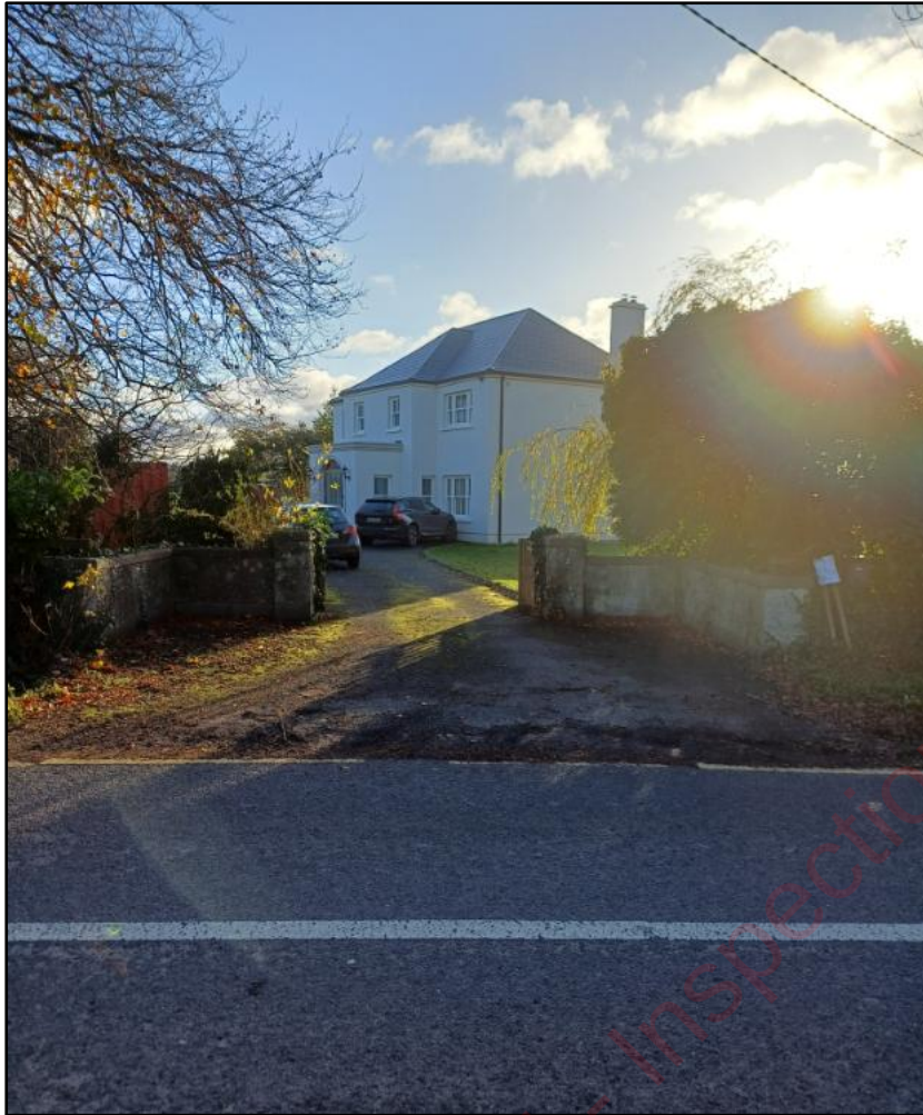
Fig 7: Site inspection photo.
